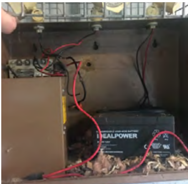
Photo 1 – Damaged Emergency Light
