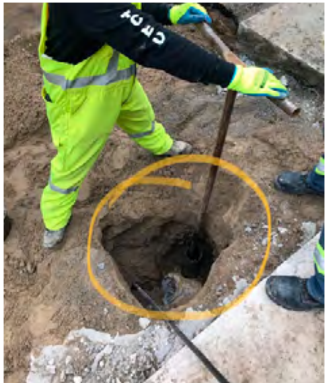
Photo 2 – Abandon underground valve >95% closed
